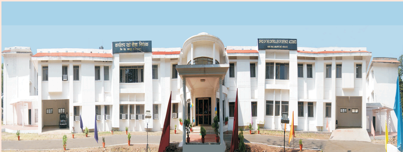
New Office Premises of CDA, Jabalpur
